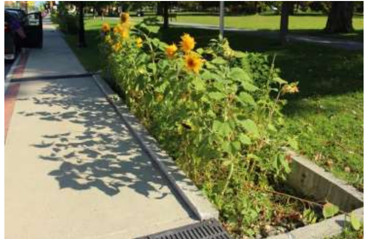
Figure 2 – Planters along Main Street beautify the area while helping collect and filter stormwater—just one way the town shows its care for the environment.
